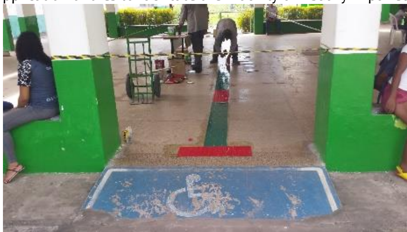
Figure 7 - Application of tiles to facilitate the mobility of visually impaired individuals.
